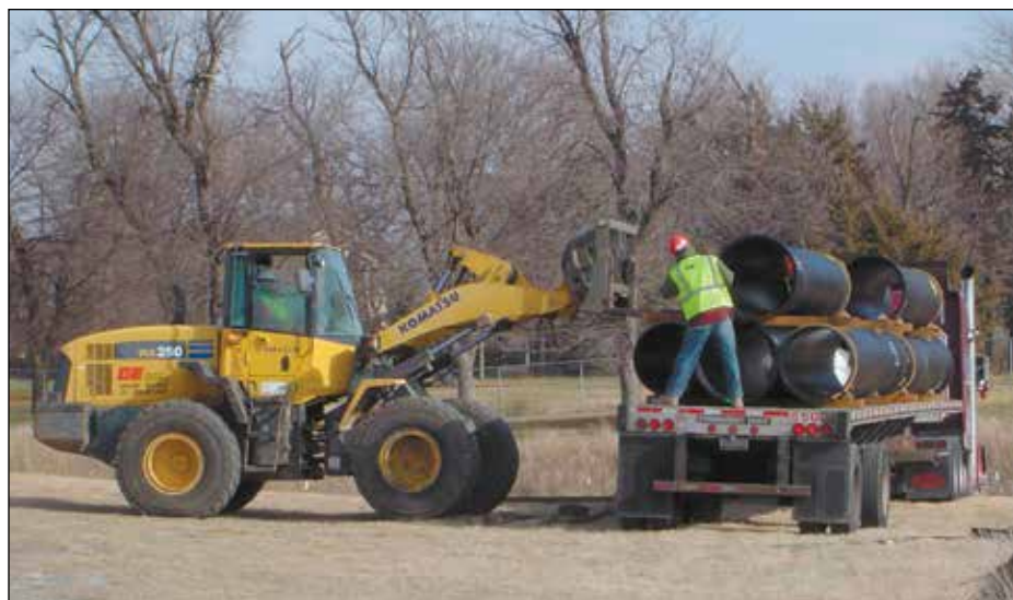
General Excavating utilized a Komatsu WA250 Wheel Loader on the project
