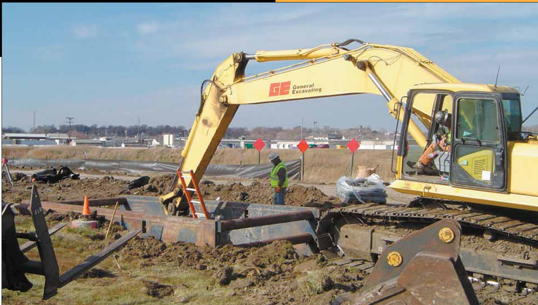
Crews dig a trench for the project's piping.
